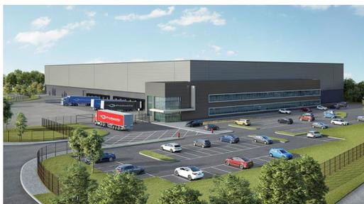
A 2022 DTZ ESG case study is the 148,240 Sq. Ft / Industrial / Distribution facility at Trafford Park, Manchester. This asset improvement scheme set to achieve BREEAM Excellent and an EPC A+ rating through the incorporation of 1,700 sq m of PV panels (generating 295,700 kWh per annum), 14 EV individual charging points, a rainwater harvesting tank and half hourly water metering and sub-metering.
